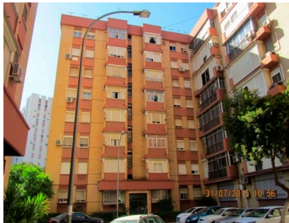
Figure 2. Northwest-facing façade of the building.
