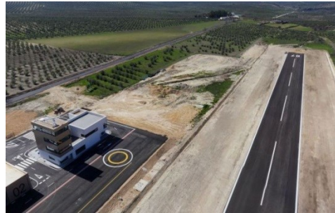
b) Outdoor flight facilities for UAVs (ATLAS Centro de Vuelos Experimentales, Jaén)
