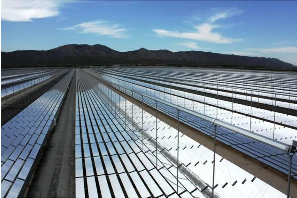
Figura 1-4 – Colector lineal Fresnel.
