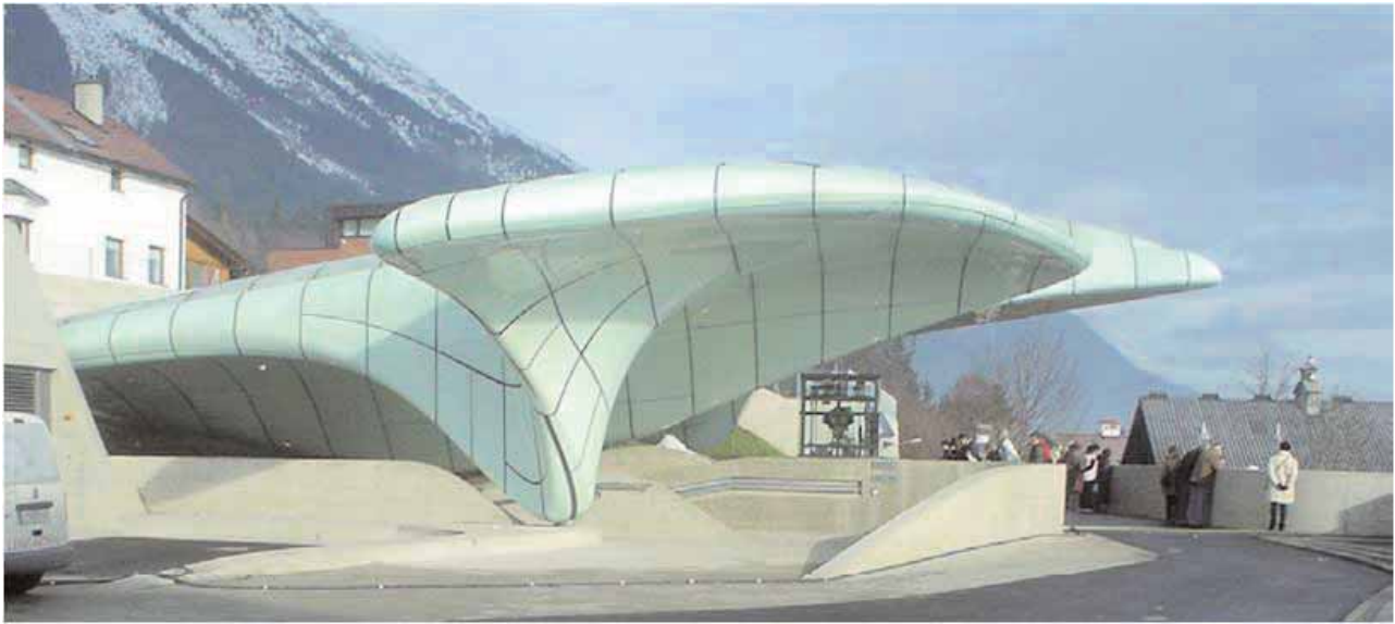
Fig. 4: Nordpark Cable Railway Station, Zaha Hadid Architects, Innsbruck, Austria, 2004-2007
