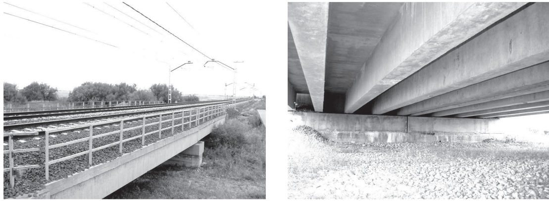
Figure 11: Railway bridge under study
