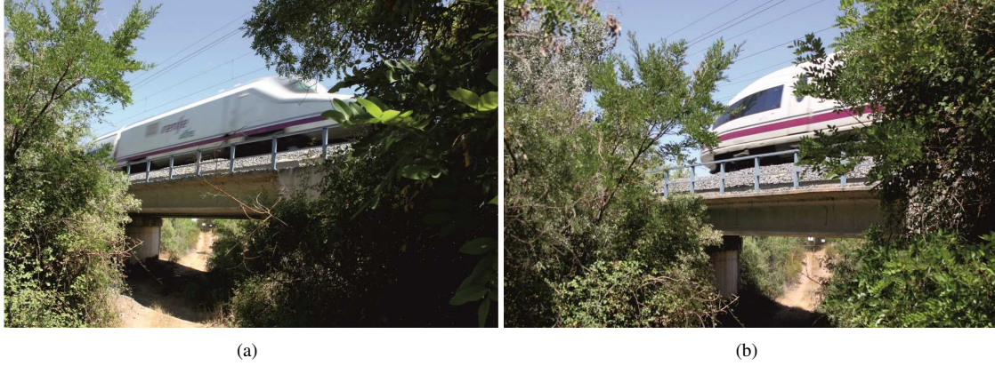
Figure 11: Arroyo Bracea I Bridge. Experimental campaign images: (a) RENFE Class 102 (Talgo 350) train passage at v = 263 km/h and (b) RENFE Class 103 (ICE 3) train passage at v = 279 km/h.
