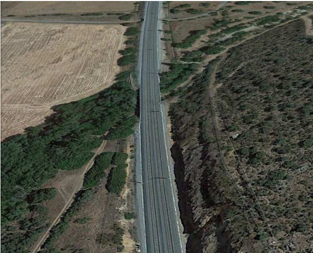
Figure 2: Arroyo Bracea I bridge (Image from Google Earth).
