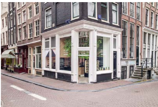
48. Standard Studio, "The Cold Pressed Juicery" -The Nine Streets, Herengracht, Amsterdam, 2016. Fachada. ((Ilust. Standard Studio_The Cold Pressed Juicery) Standad Studio. Foto: Wouter van der Sar )
