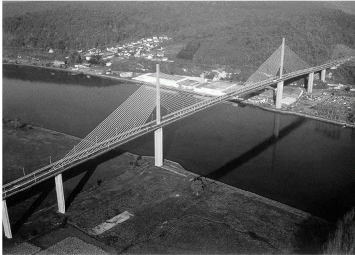
Figura 1.1. Puente de Brotonne (Finley Engineering Group , 2017)
