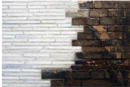
Fig. 10 Bricks 36 mm high and lengths up to 520 mm and light gray neutral (Claudio_este).
