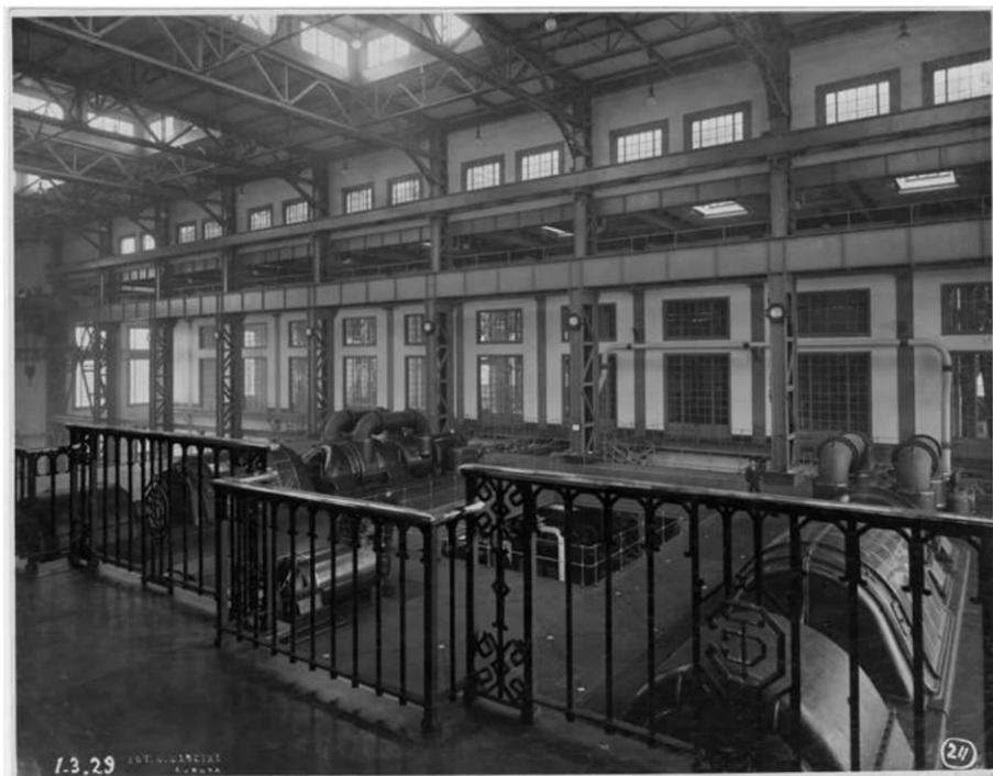
Fig. 7 Interior Sala turbinas 1927
