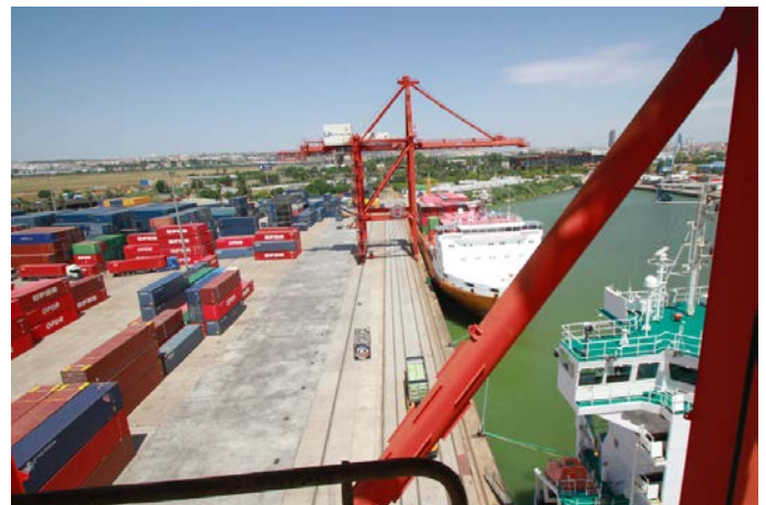
Figure 1. Partial view of the container yard in the “Batan” dock at the Port of Seville.
