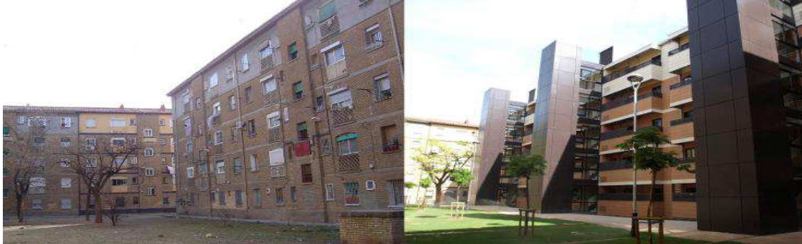
Fig. 4 "Building before and after rehabilitation". Source: S.M.R.U.Z.
