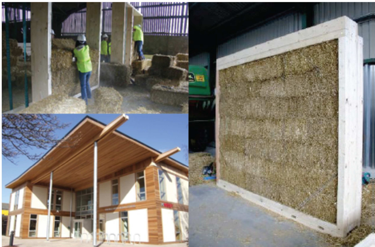
Fig.8 "Modcell, UK, prefabricated modules up to 3x3m" Source: www.modcell.com
