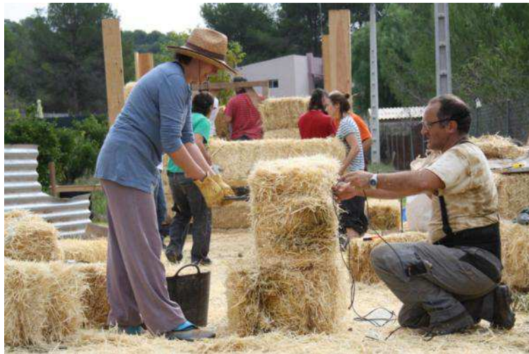
Fig.7 “Handling of Straw Bales for a load bearing Building” Source: okambuva.coop
