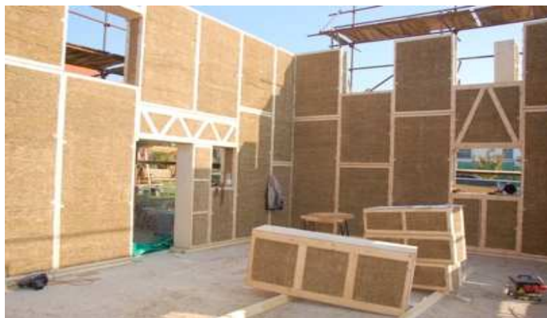
Fig.12 "Mounting walls for a house" Source: ecococon.lt
