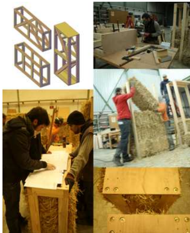
Fig.10 "Mounting modules alfaWALL" Source: okambuva.coop
