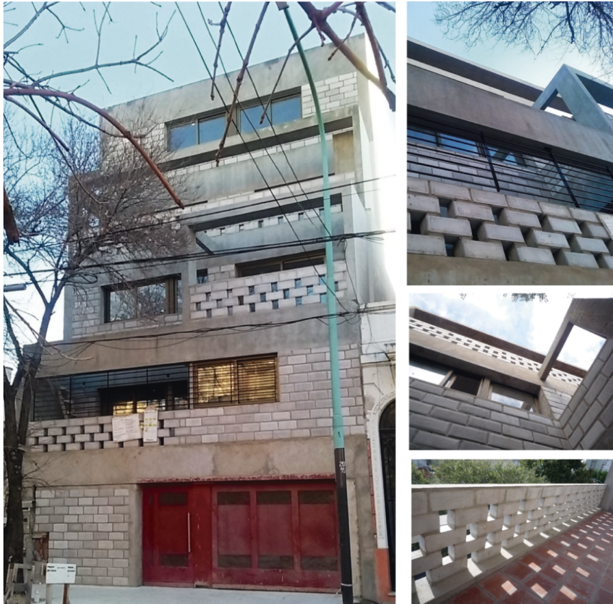
Fig. 1 Exteriors and balconies. Source: own elaboration
