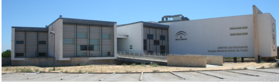
Fig. 2 Visitor Centre's general view
