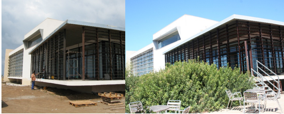
Fig. 7 Use of Corten steel. The photograph on the left is taken during the execution of the work in 2006. The image right on a visit in August 2016
