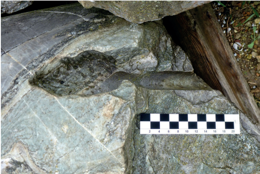
Fig. 5. Cavity for marble patch in the finish of a metal spike.
