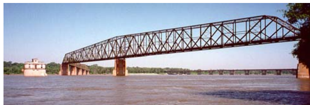
Figure 4.7: Chain of Rock Bridge. Source: astro4.ast.vill.edu
