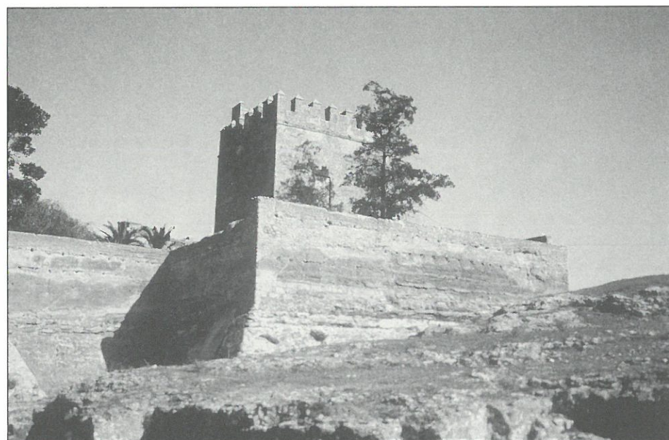
Plate 7. Mairena del Alcor outer wall, dating from the 15th century.
