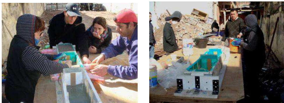
Fig.6 On-site training work. Source: own elaboration
