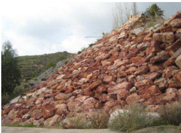
Fig 6 “Deficient breakwater wall” and Fig 7 “Ground movement and sliding wall”
