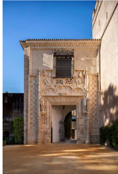
Figure 3. Marchena facade in the Real Alcázar of Seville. In the restoration, previously the cleaning process and structural consolidation is performed, lime mortar is applied in stone joints, stone mortar and stone recomposition, and finally the masonry and stone sculptures were protected and consolidated with thin layers of lime mortars.
