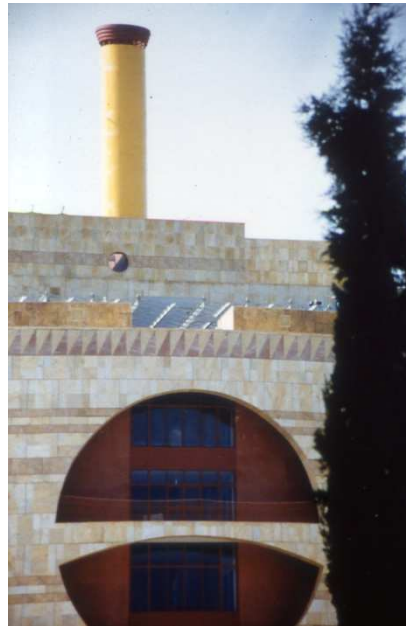
Figure 5. Torre Triana building. Architect Francisco Javier Sáenz de Oiza. Stucco coating
