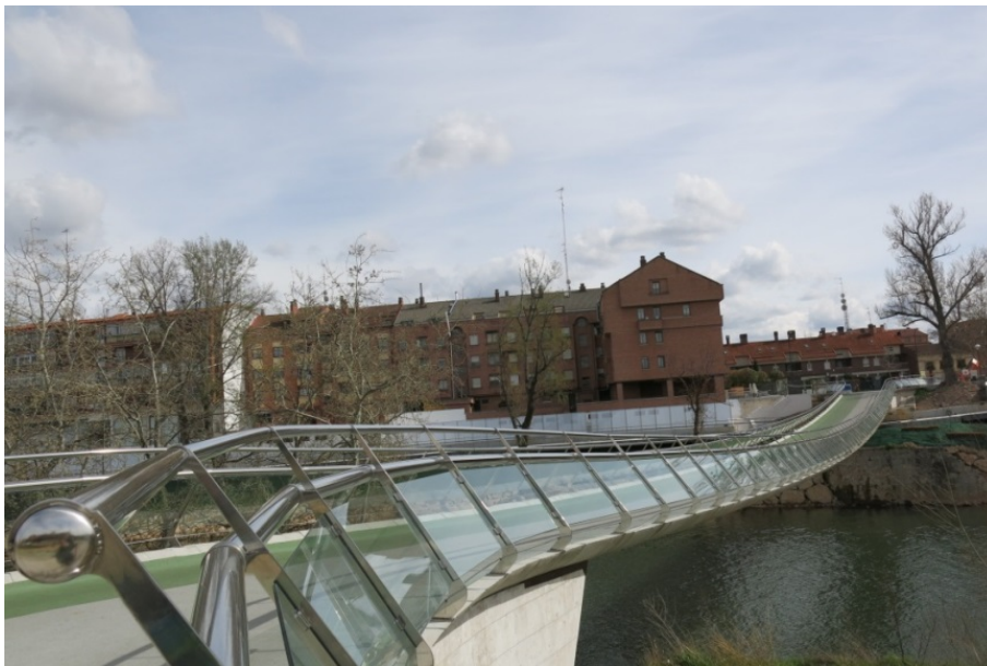
Figure 1. Stress ribbon footbridge under study
