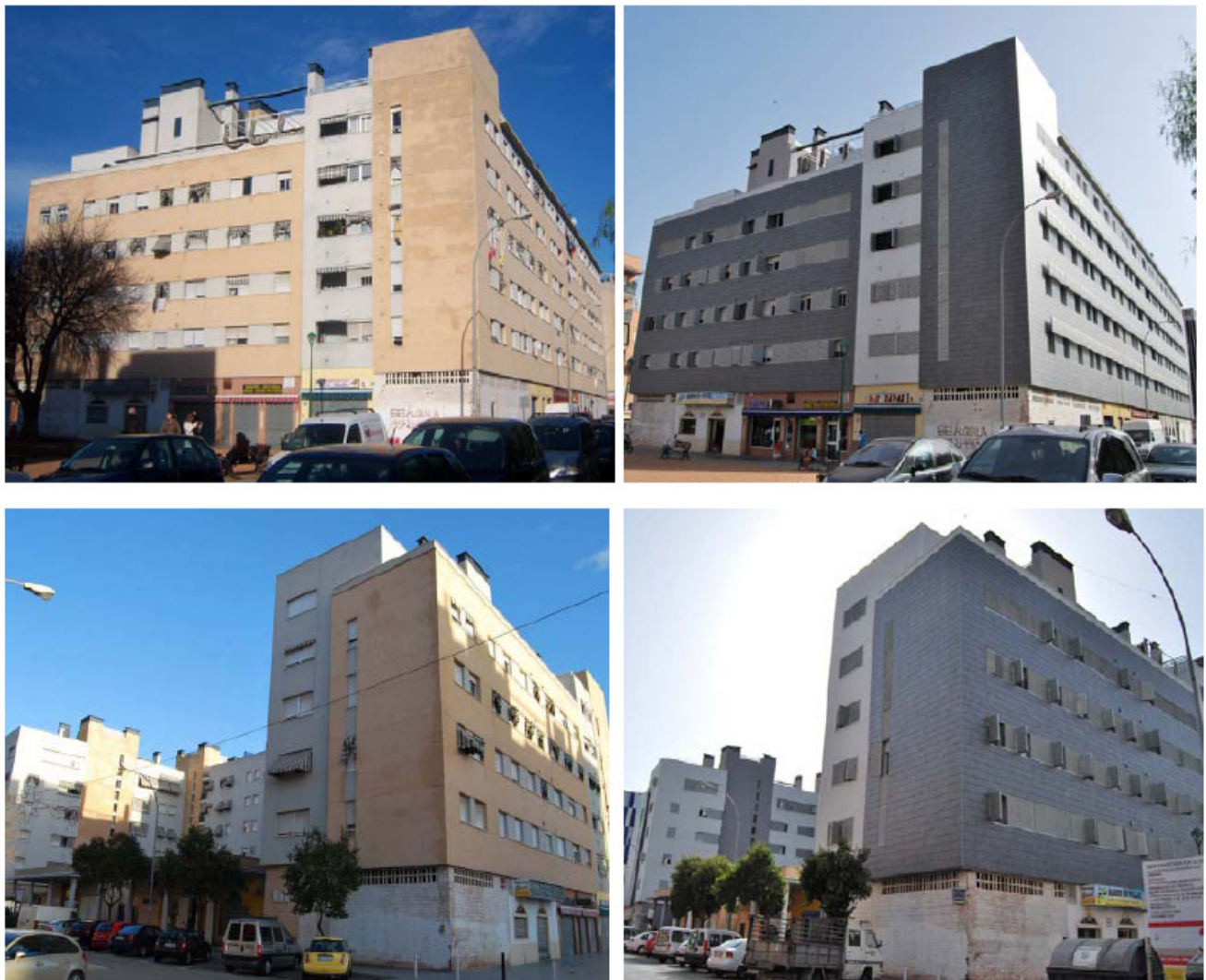
Figure 2. Building in original condition (left) and following retrofit (right).
