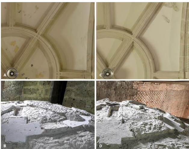
Fig. 11: Detail of vault AC13: (a) intrados and (b) extrados. Detail of vault CE57: (c) intrados and (d) extrados
