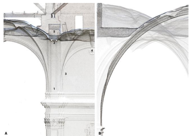
Fig. 14: (a) Transverse rib non distorted (1-2), wall rib distorted (3-4), and voussoir on top of the keystone of a transverse rib (5). (b) Hollowed out diagonal ribs and low wall on the haunches
