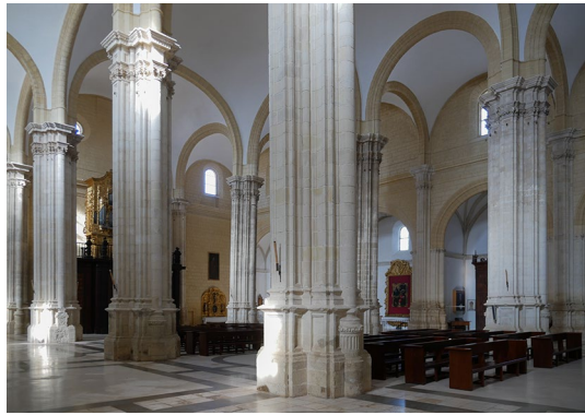
Fig. 2 Nave and aisles section of the collegiate church of Osuna
