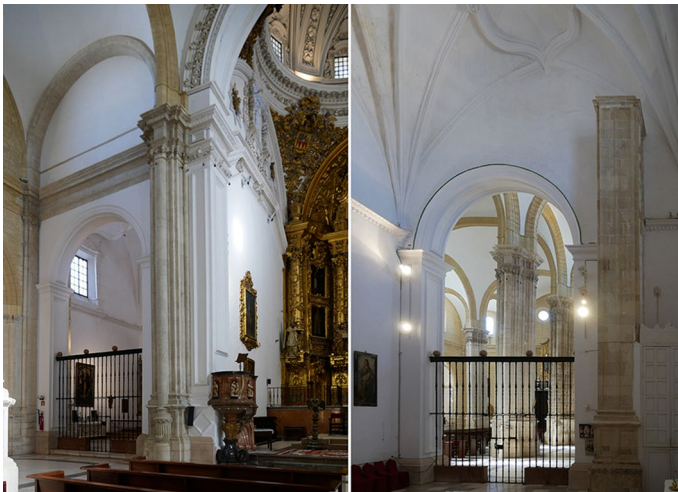
Fig. 5 North chapel of the apse of the collegiate church of Osuña: entrance arch and interior
