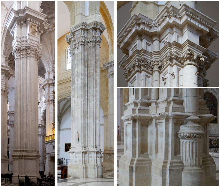
Fig. 14 Pier in Granada Cathedral (left) and pier in the collegiate church of Osuna (general and details)
