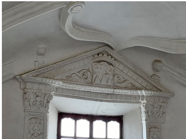
Fig. 13 Renaissance ornamentation on the window of the north chapel of the apse, with the ducal coat-of-arms, overlaying the wall arch of the vault
