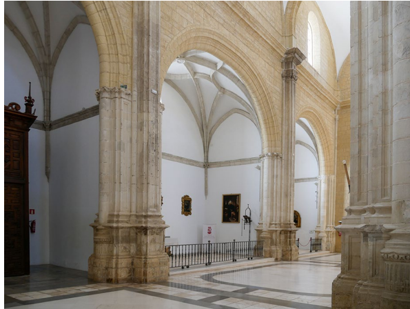
Fig. 17 Side chapels and south aisle of the collegiate church of Osuna
