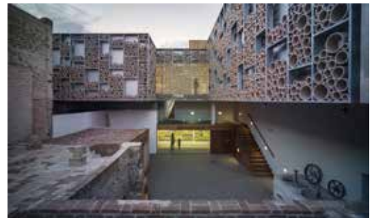
Figure 8. Image of the courtyard. Author: © Jesús Granada, 2013. Source: AF6 ARQUITECTURA.
