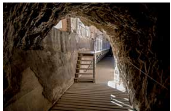
Figure 8. View of the tunnel. Author: Jesús Ponce. Source: Luis Machuca y Asociados, S.L.P.
