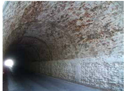
Figure 11. Gorgoracha Tunnel, Granada (1848).
