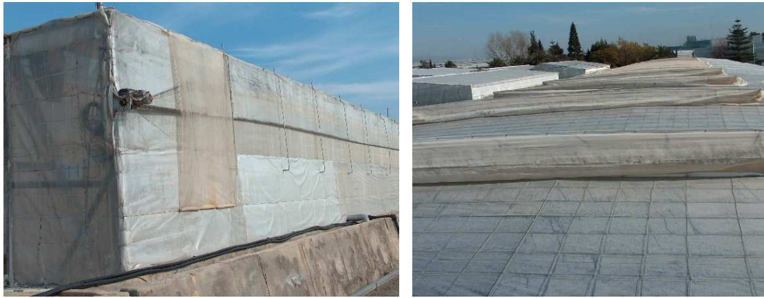
Figure 3.24: View on the lateral (left) and roof (right) windows of the experimental greenhouse.
