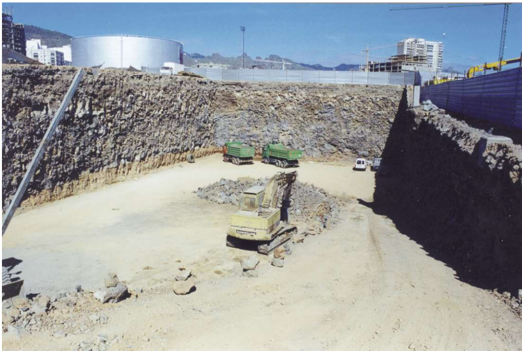
Figure 2. Front of the 17.5 m deep excavation
