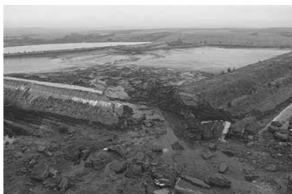
Figure 1. Ajkai Timfoldgyar dam failure.
