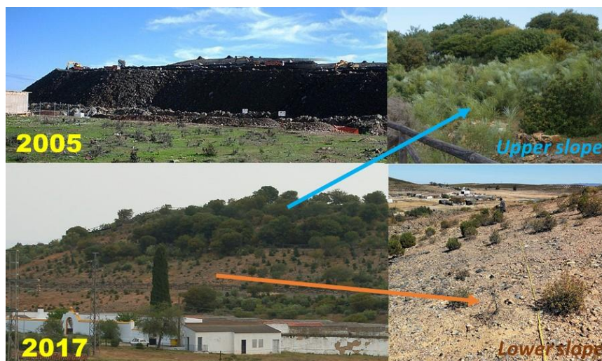
Fig. 5. General view of the waste rock pile from the town of Tharsis; in 2005, when the rehabilitation started (left top), and in 2017, once covered by vegetation (left bottom). The contrast between revegetated plots at the upper slope (right top) and the barren soils at the lower slope (right bottom), affected by the acid mine drainage. Photos by EGMASA (2005 picture) and T. Marañón
