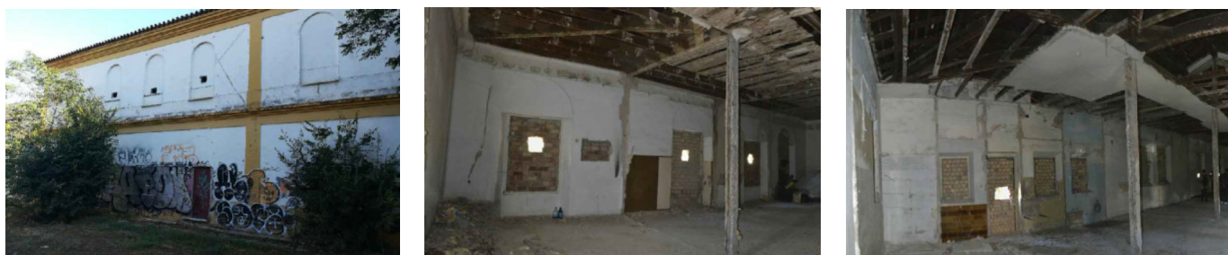
Figure 2. Current-state pictures of the studied building.
