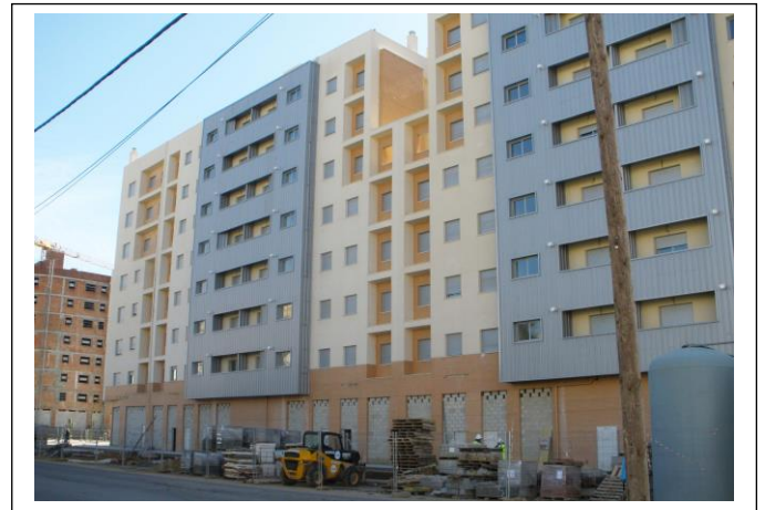
Figure 5. External views of the M.C.-1.2 perimeter block building, during its construction
