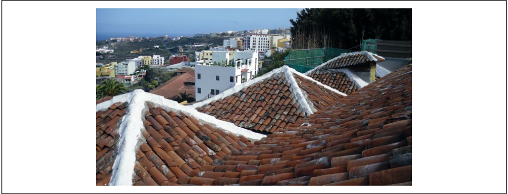
Figure 7. The church of Saint Marcos in Tenerife, Canary Islands (Spain). Exterior view of the sky-light constructed over one of the lateral chapels.
