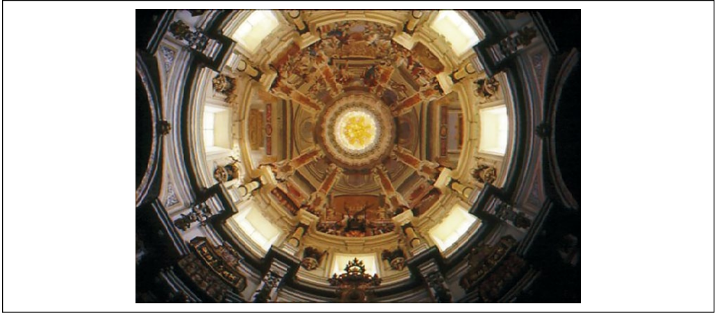
Figure 1. Interior of the church of Saint Louis of the Frenchmen, Seville, Spain. Source: Jose M Almodovar-Melendo.
