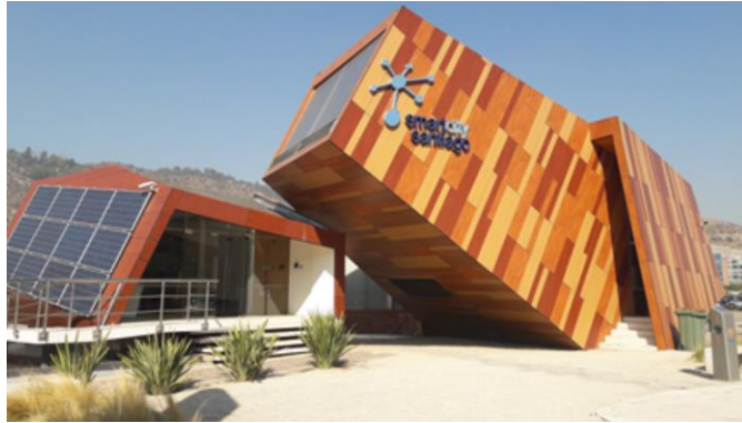
Fig. 3. Enel Smart Grid Building (Santiago de Chile, Chile)
