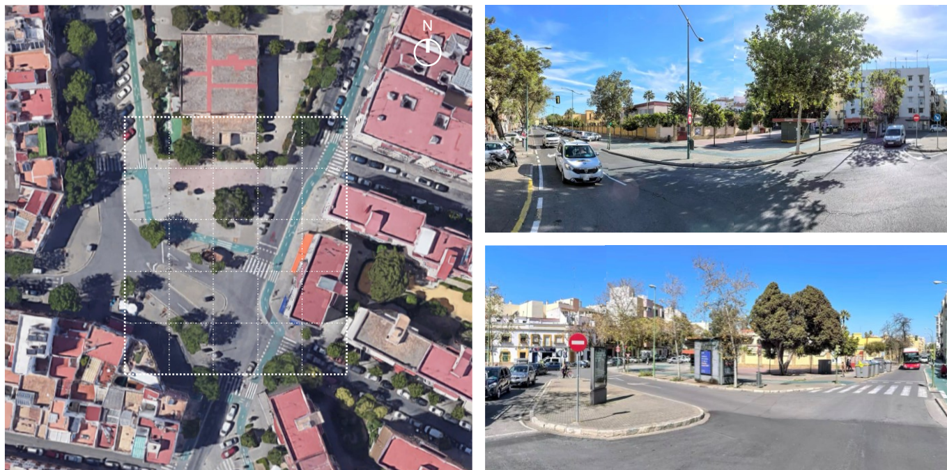
202 203 204 Figure 2. Square before renovation 205
