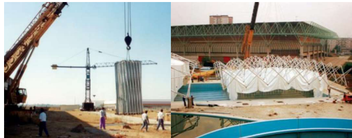
Fig. 6. (Left figure) Test of the deployment process; (Right figure) Deployment process in the olympic pool.
