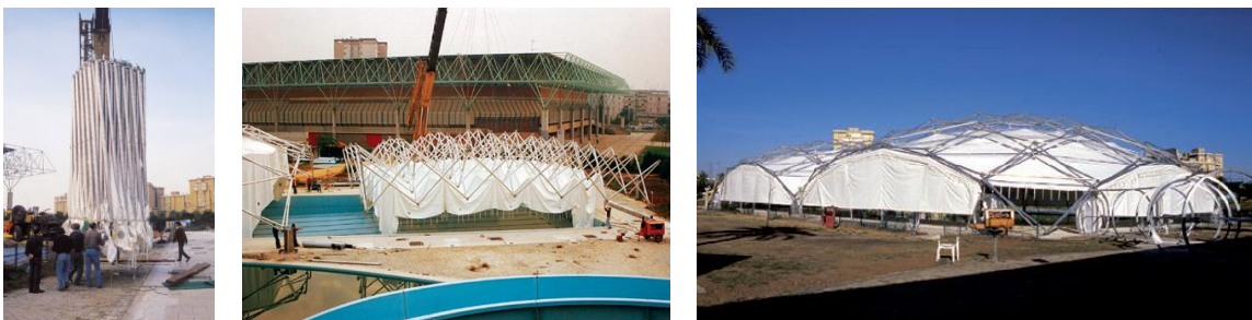
135 136 Fig. 7. Gravity deployment system in San Pablo pool (Seville).
