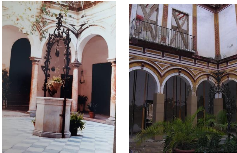
Figure 1. View of the courtyard of the Arizón Palace: a) Photograph of the Courtyard of Honour in 1989 and detail of the central well; and b) Photograph of the Courtyard of Honour in 2009 at the beginning of the last rehabilitation.
