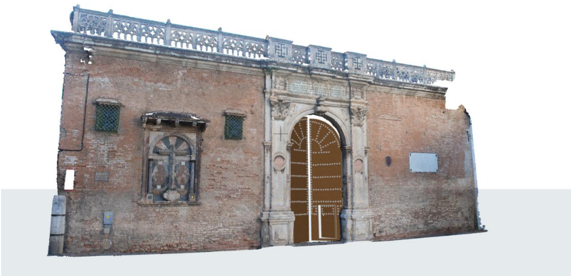
521 Figure 22. Global point cloud of the façade and BIM of the door.
