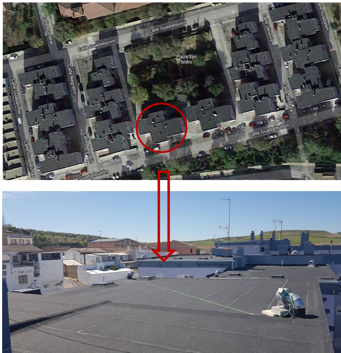
Figure 17. Condition of the district after renovation
