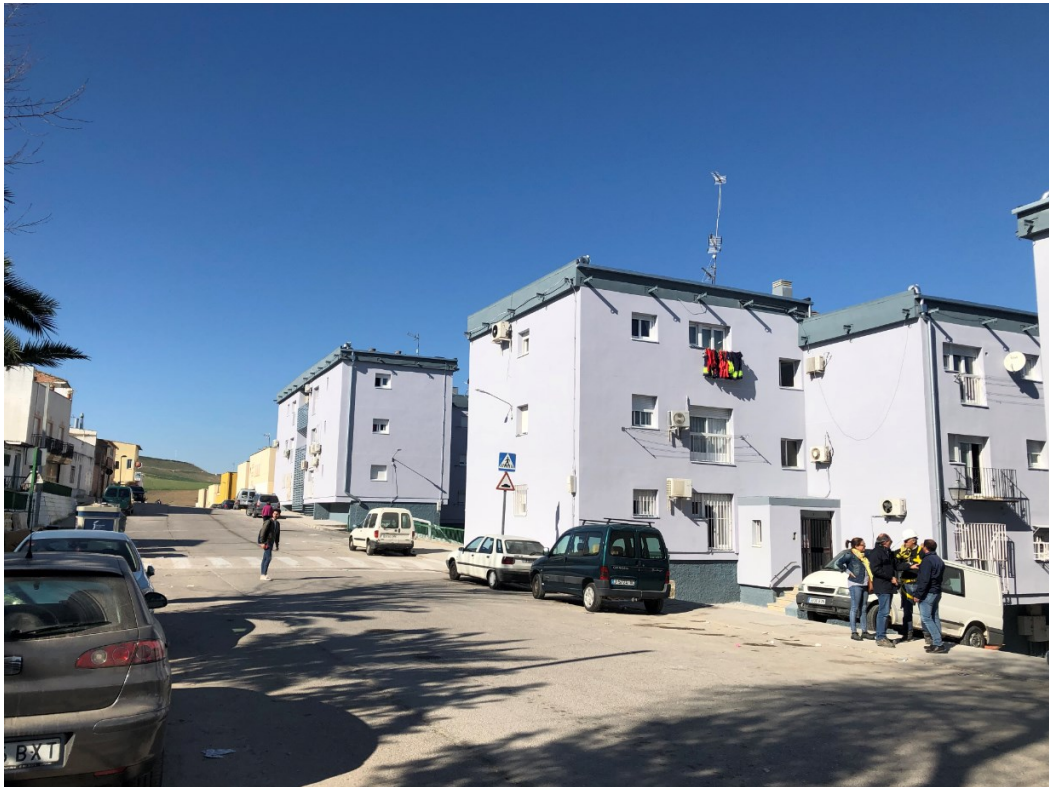
Figure 11. Condition of the district after renovation
