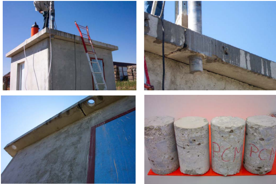
Figure 2. Concrete test samples extracted from both cubicles
