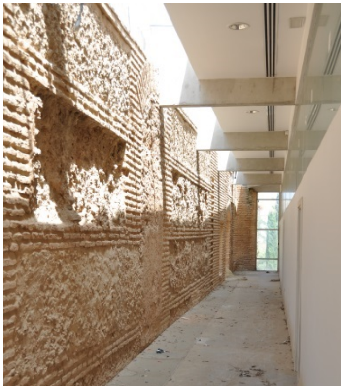
Figure 5. View of the new construction. Upper floor.
