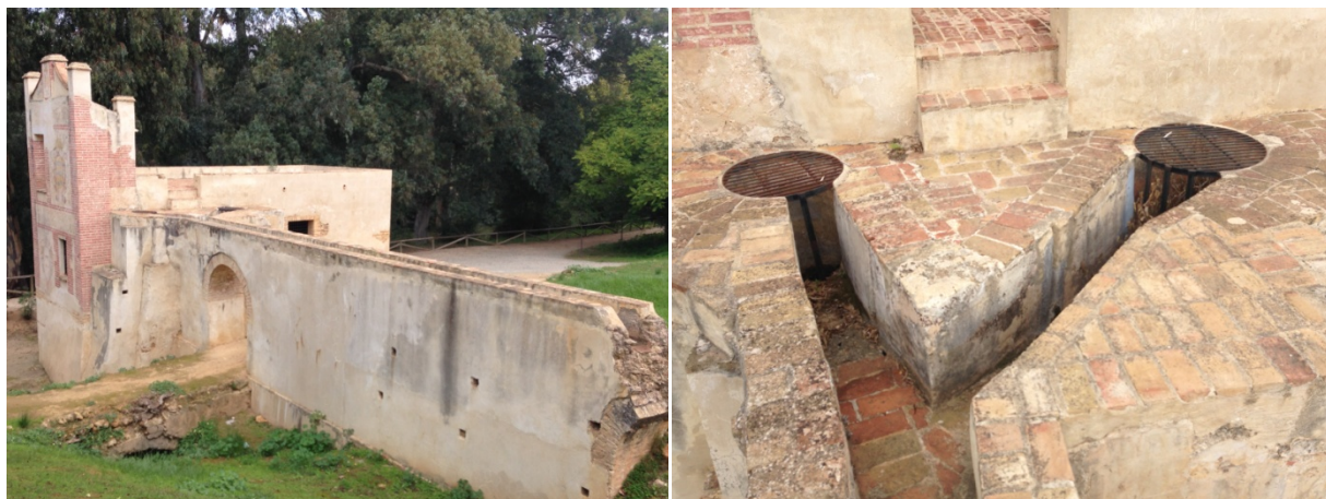
Figure 8. Penstock mill called La Tapada , Alcalá de Guadaíra
