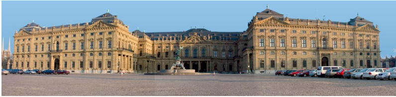
Fig. 1 Front of the Würzburg Residence (Germany).
