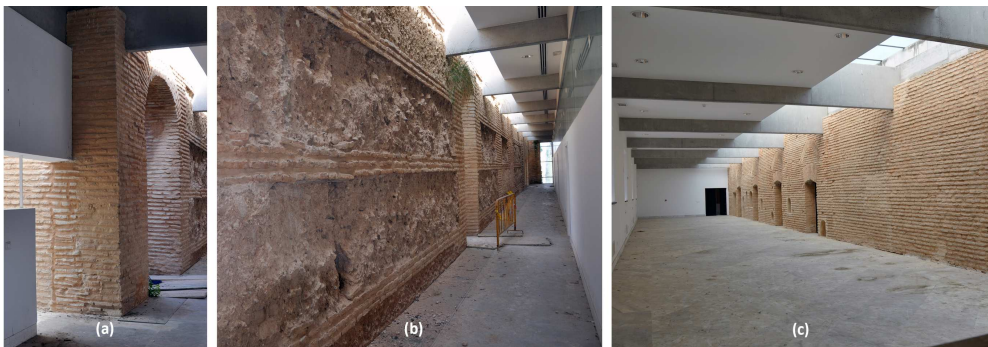
Figure 5: New building structure: (a) resting on the ancient one; (b) east wing; and (c) south wing.
