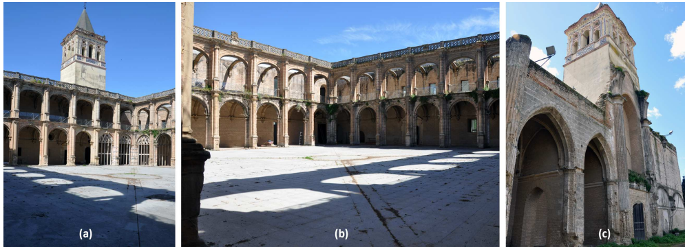
Figure 1: Views of the current state of the Monastery of San Jerónimo de Buenavista, Seville, Spain: (a) North and East wings and tower; (b) South and East wings; and (c) remains of the cloister church and the tower.
