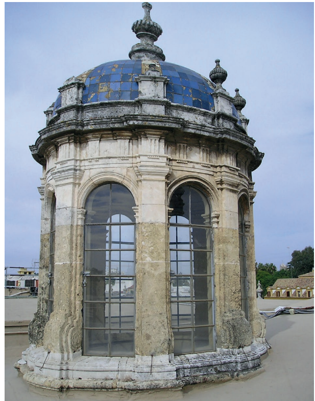
Fig. 3c. Lanterns designed by Sebastián Van der Borch for light entry into the manufacturing plant. Source: Authors' own creation.
