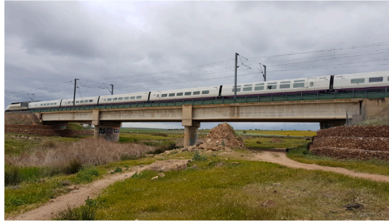
Fig. 3. HSL bridge over Jabalón river (38°53'51.3"N 3°57'53.0"W).
