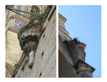
Fig. 8: Left: corbel in the choir loft; right: tas-de-charge over one of the pilaster capitals
