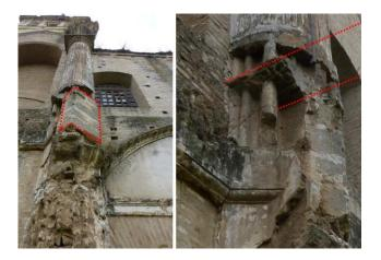
Fig. 9: Joint between the mouldings on the choir front and the vault with the pilaster
